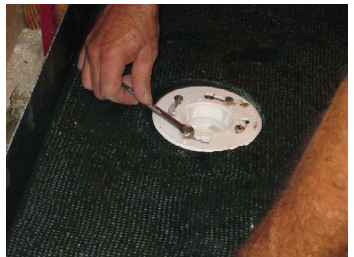
Step 4 Clamp Shower Base To Drain
