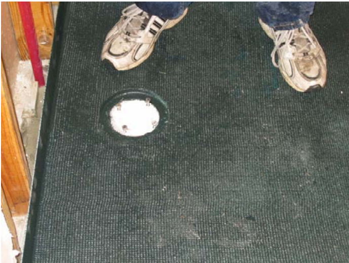
Step 3 Ensure That Shower Base Is Firmly Set
