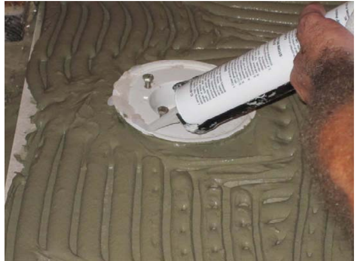
Step 2 Place Silicone On Perimeter Of Drain
