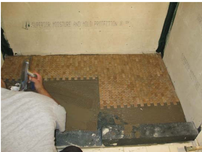
Step 5 Trowel Thin-Set & Install Tile As Usual
